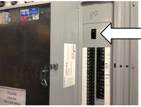
Main power switch for the fuse boxes. There are three boxes, pull whichever is needed
